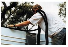
Gluing Presstite to top rim of tank
